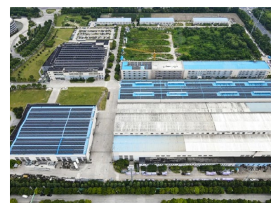
The headquarters park features a 3.1 MW distributed photovoltaic system installed on the rooftops
